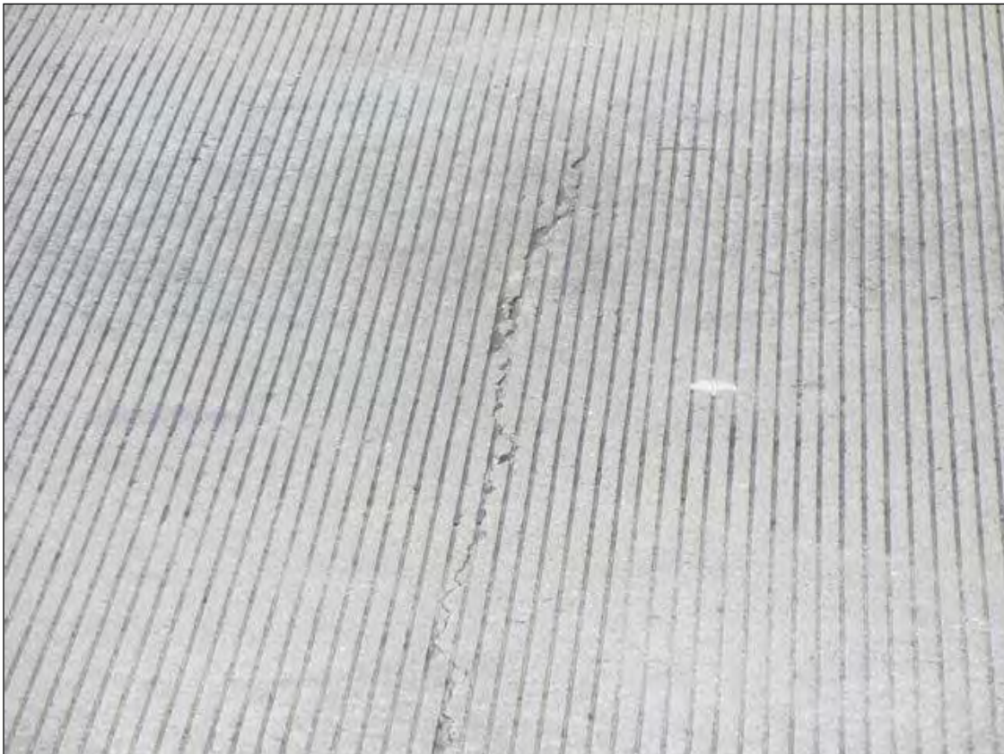
TRANSVERSE CRACKS IN ALL SPANS
