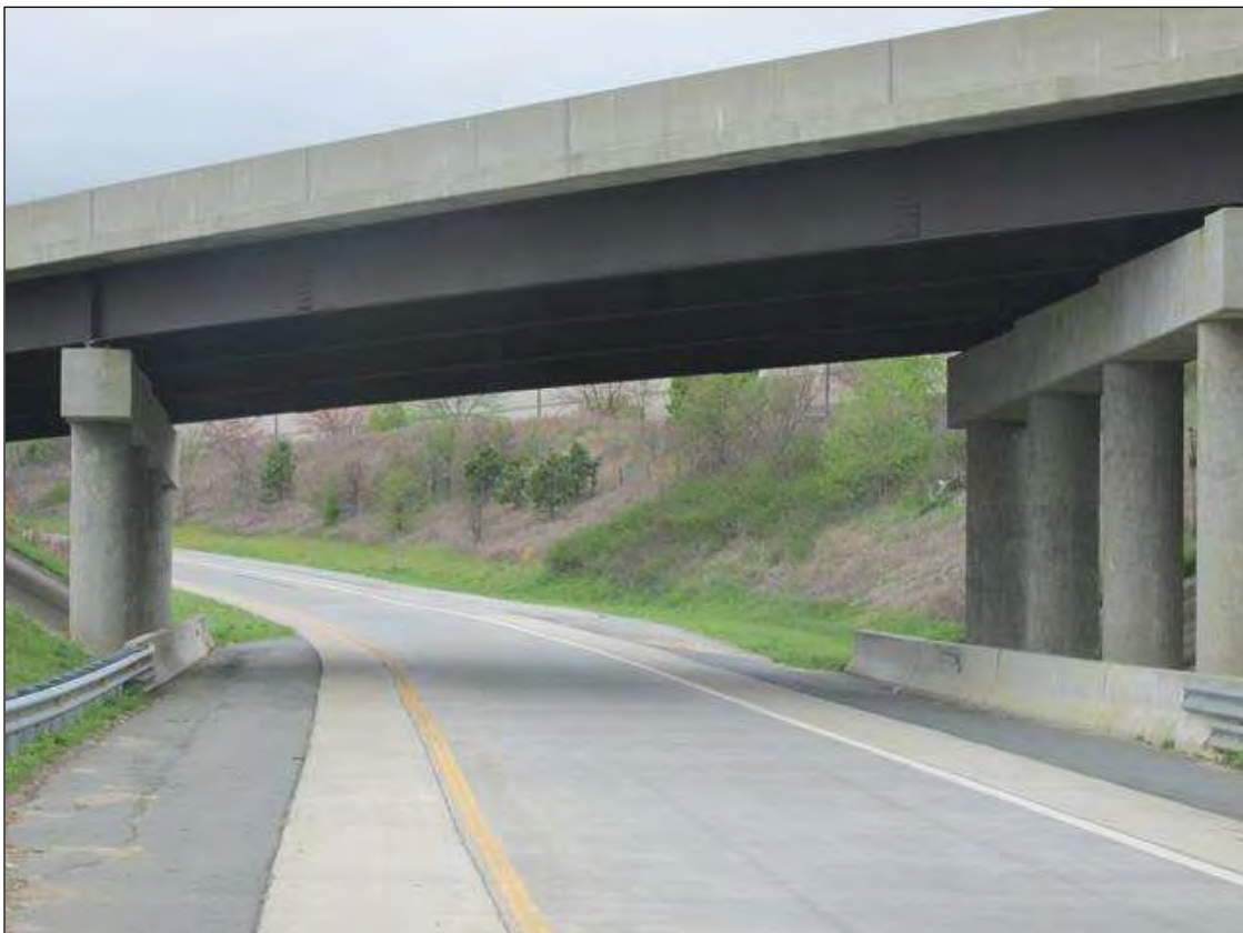
NORTH OPENING, SPAN 2
