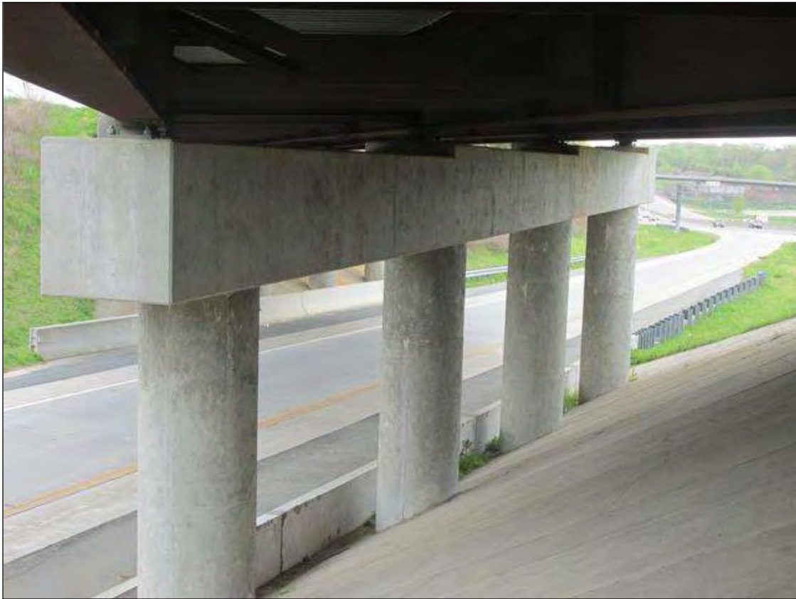
PIER 1 LOOKING EAST
