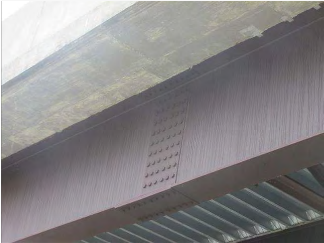
SPLICE PLATES IN SPAN 2
