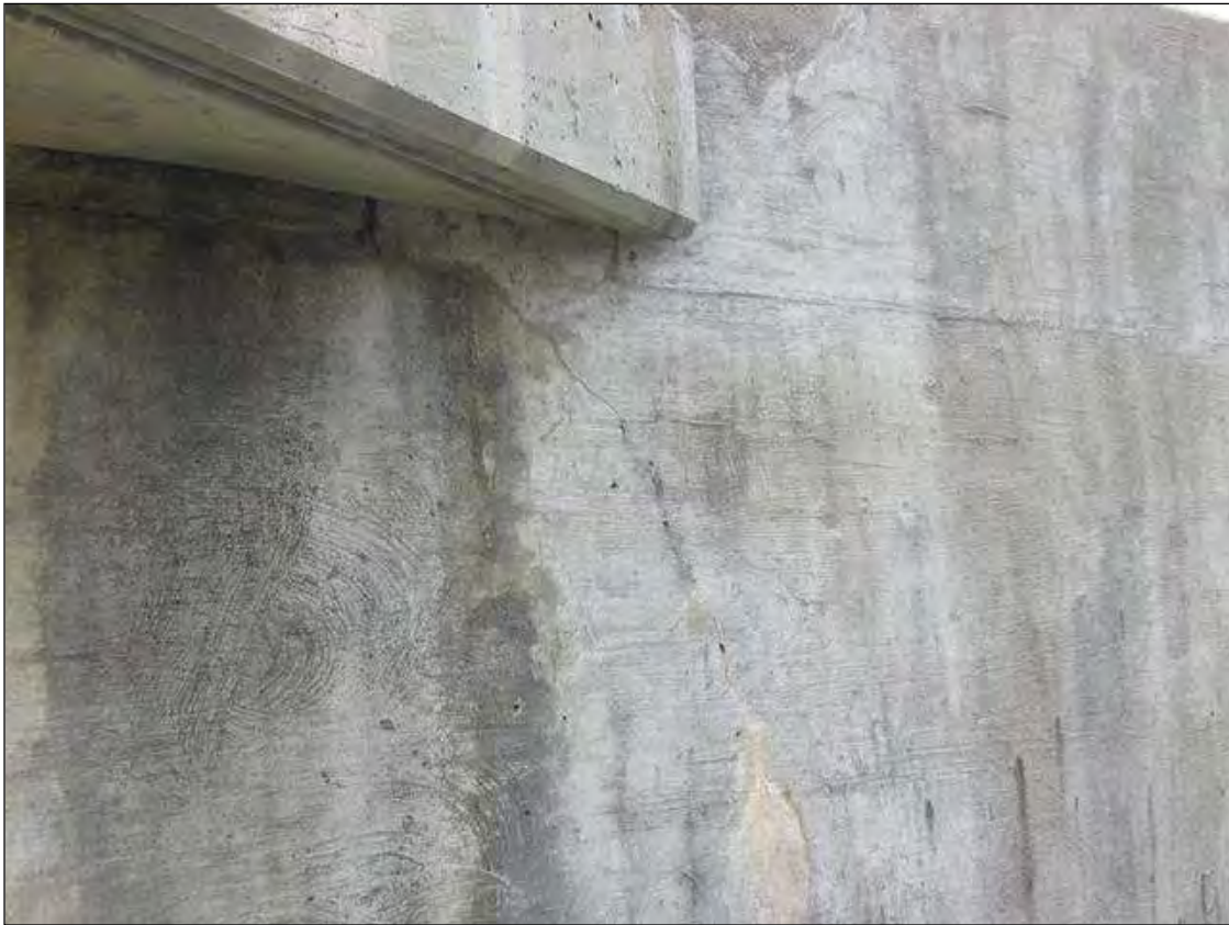
HL. DIAGONAL CRACKS IN BOTH ABUTMENT BACKWALLS
