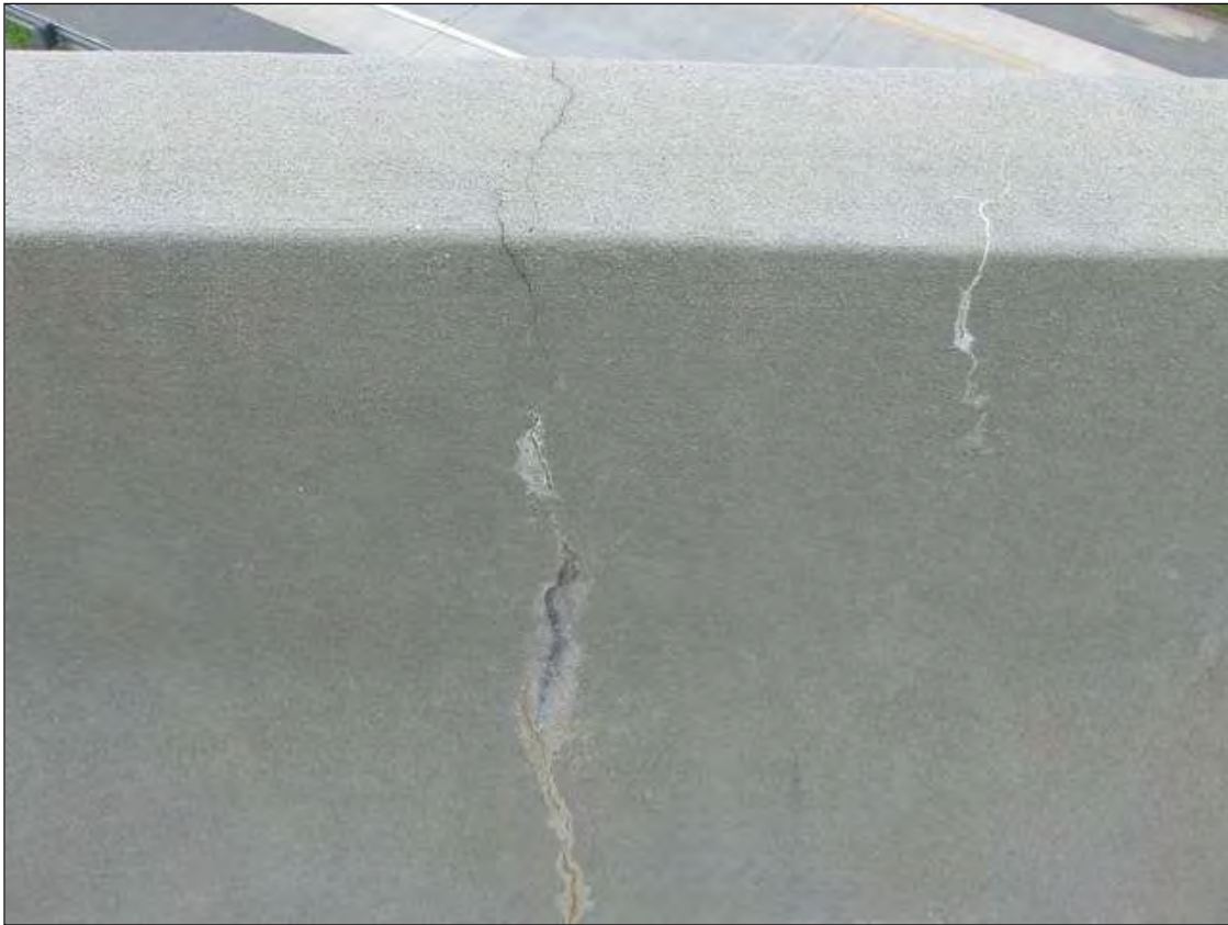
CRACKS IN BOTH RAILS
