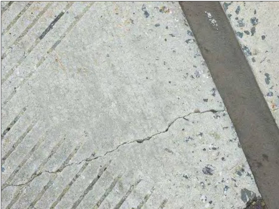
CRACKS IN THE SPAN ENDS
