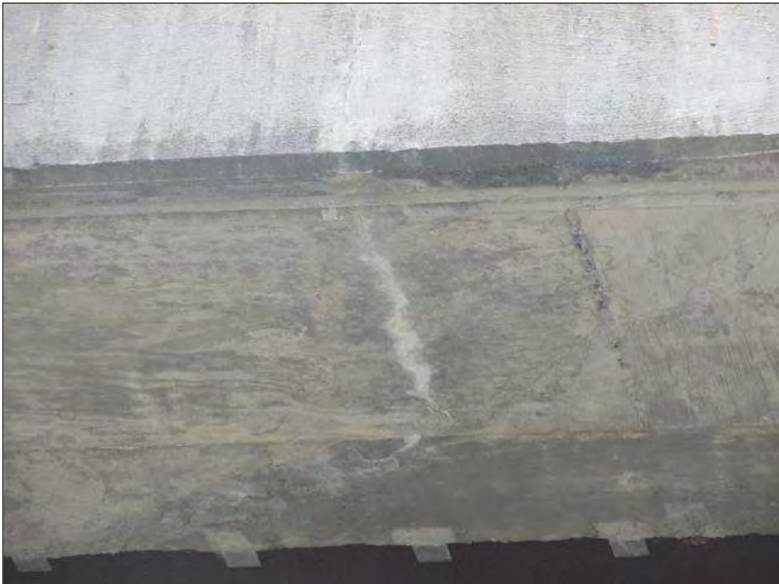
CRACKS IN BOTH OVERHANGS
