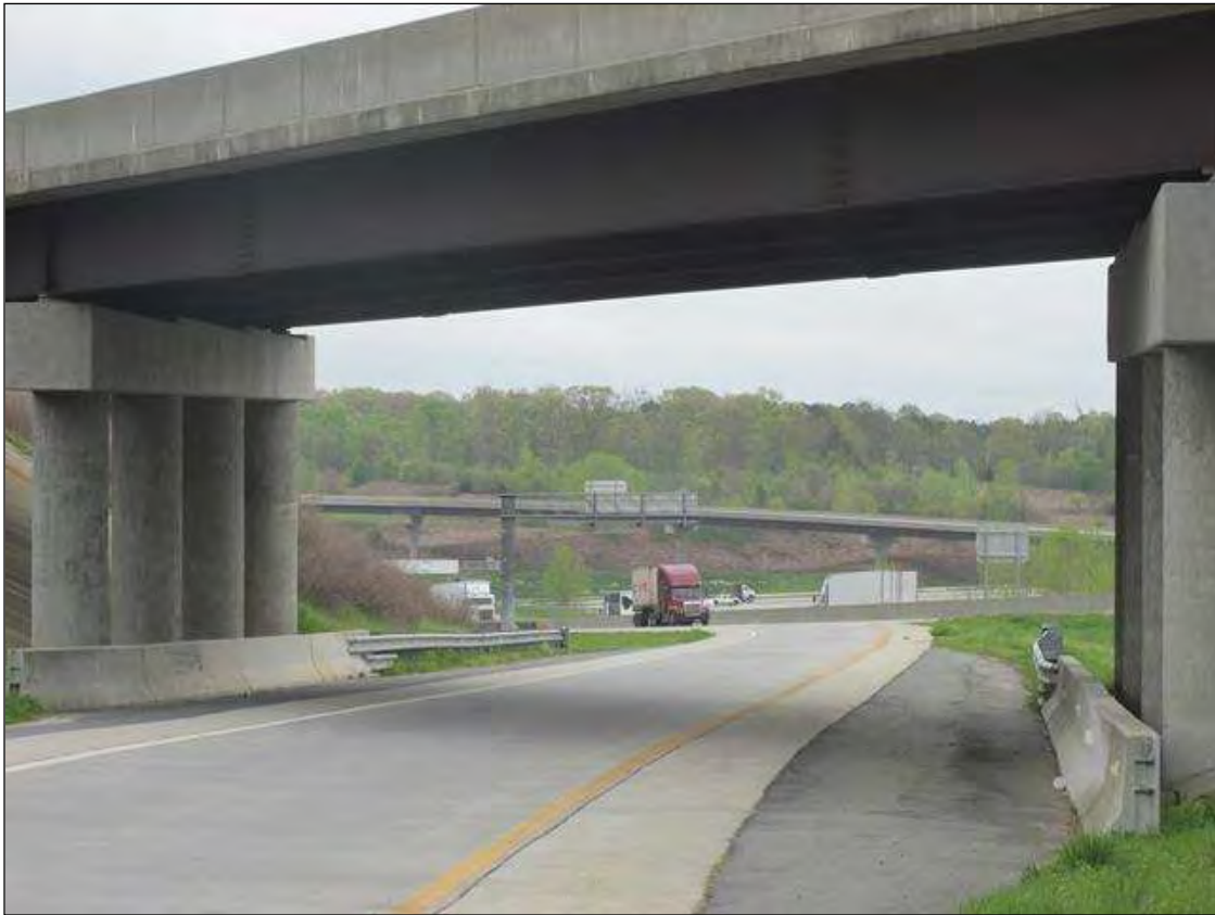
SOUTH OPENING, SPAN 2
