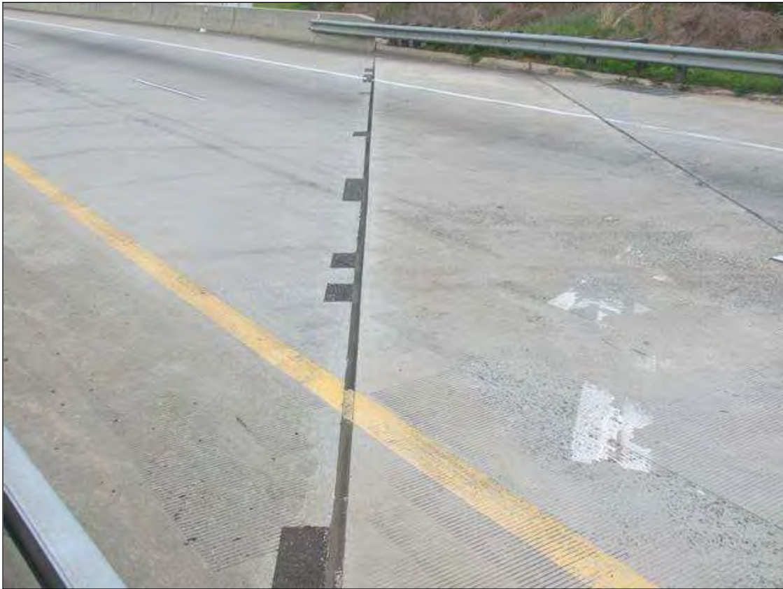
EXPANSION JOINTS AT BOTH ABUTMENTS
