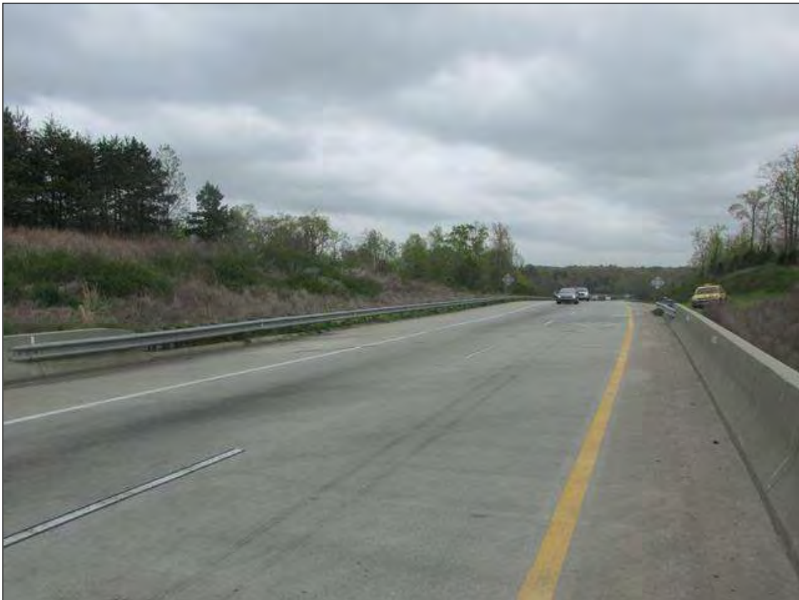
GUARD RAIL LOOKING EAST
