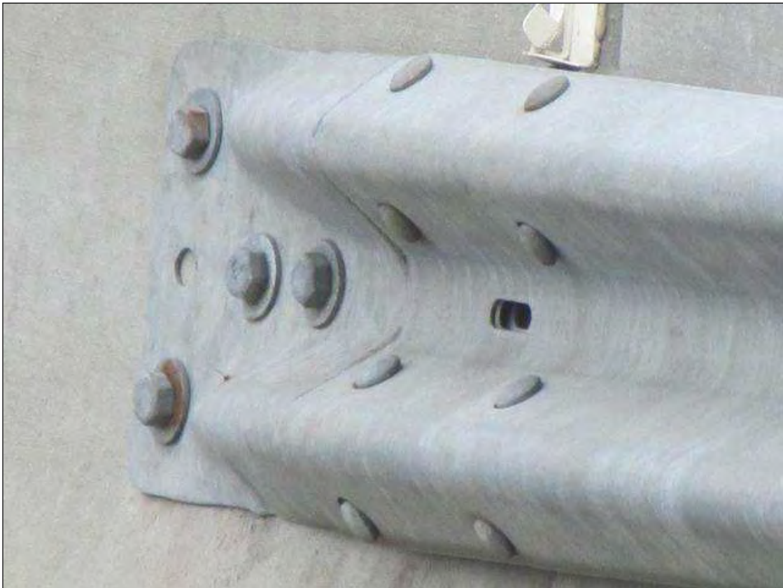
GUARD RAIL CONNECTION NE CORNER ALL SIMILAR
