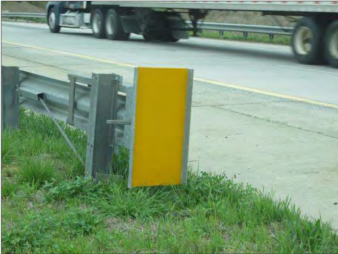
GUARD RAIL TERMINAL END AT THE SE END ALL SIMILAR
