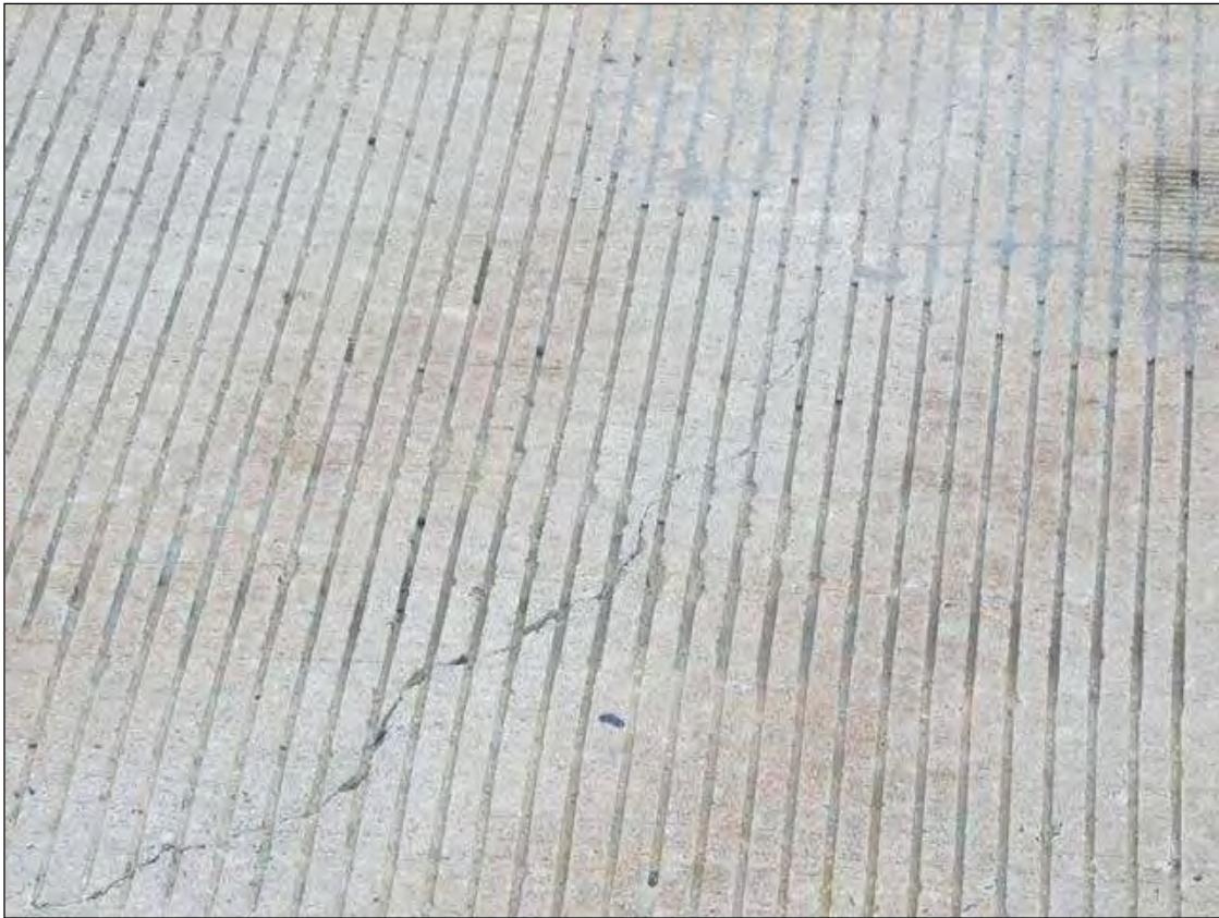
HL. TRANSVERSE CRACKS IN BOTH APPROACH SLABS
